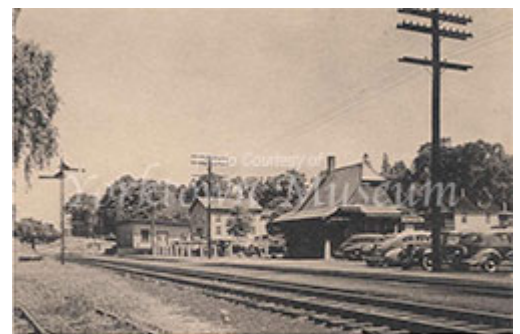
Railroad Station and stores c. 1938 Courtesy of Yorktown Museum
