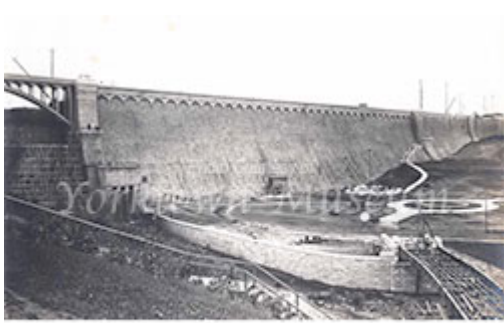
Construction of the New Croton Dam c. 1902 Courtesy of Yorktown Museum
